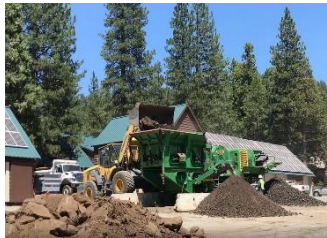
Rock Crushing-Used Native Material for Backfill
