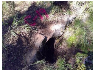
C-19 Culvert Before
