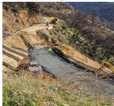
Mechanical Stabilized Earth Walls Site 1 before, in progress, and complete.
